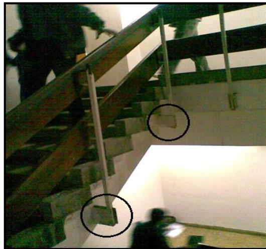
Figure 4. 5: Picture showing connection on edges of stairs
