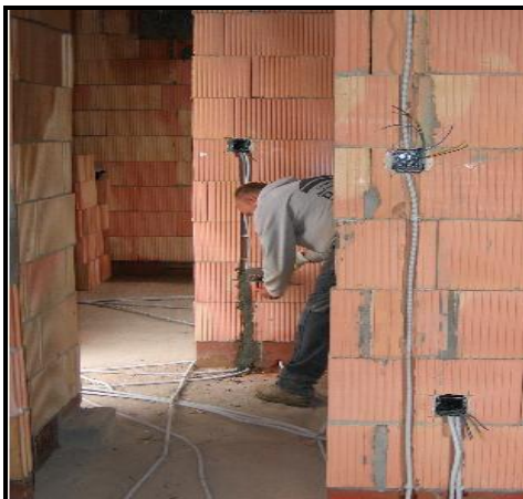
Figure 4. 6: Picture showing worker during electrical installations
