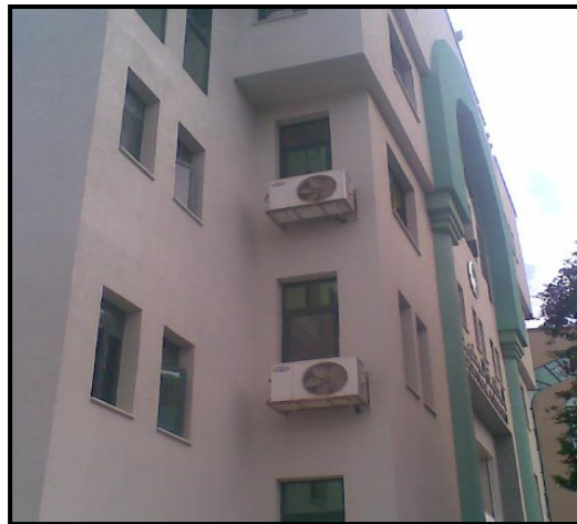
Figure 4. 11: Picture showing split unit placed near a window
