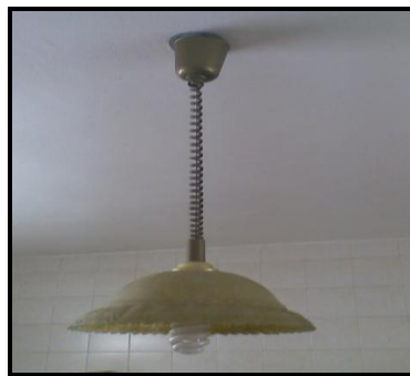
Figure 4. 9: Picture showing light fitting that could be lowered
